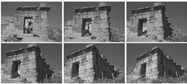
Figure 2: Image sequence which was used to build a 3D model of the corner of the Roman baths
