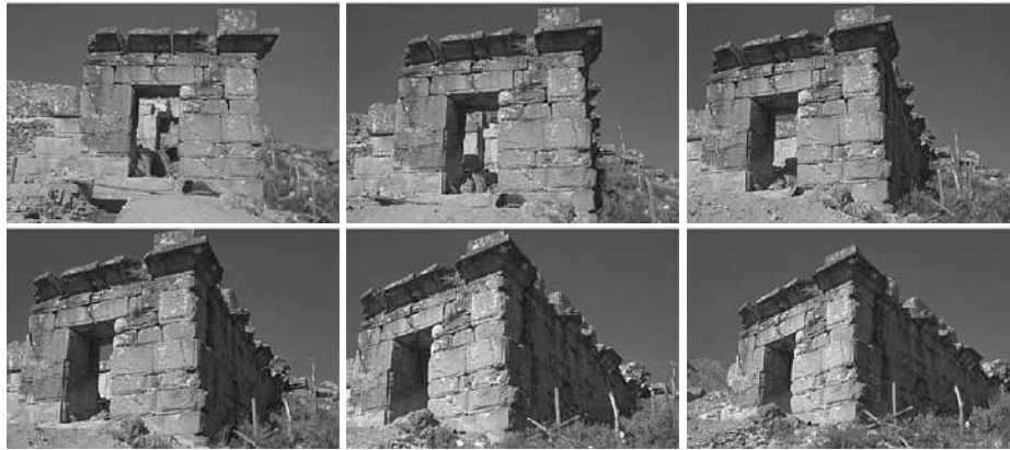
Fig. 12. Image sequence which was used to build a 3D model of the corner of the Roman baths.
