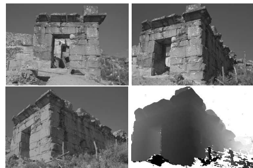
Figure 12. Images 1, 3 and 6 of Roman Bath sequence. Lower right: estimated depth map (dark = near, light = far).
