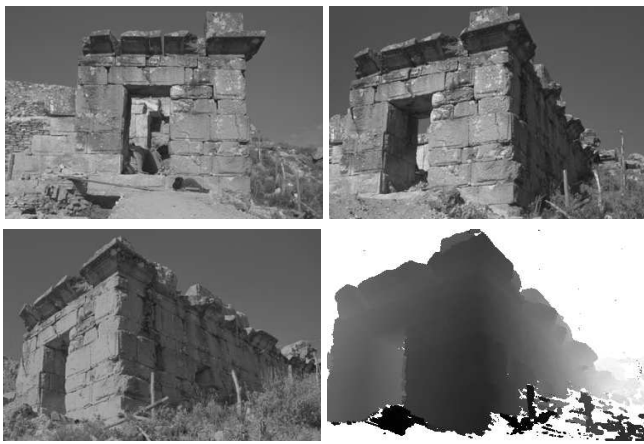
Figure 8. Images 1, 3 and 6 of Roman Bath sequence. Lower right: estimated depth map (dark = near, light = far).
