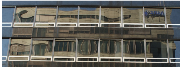
Figure 1. Real-world glass reflection. Notice that reflection in different windows on the same facade can appear very different due to minor deformations and normal variations. Our goal is to capture normal maps of real windows to faithfully reproduce this effect.
